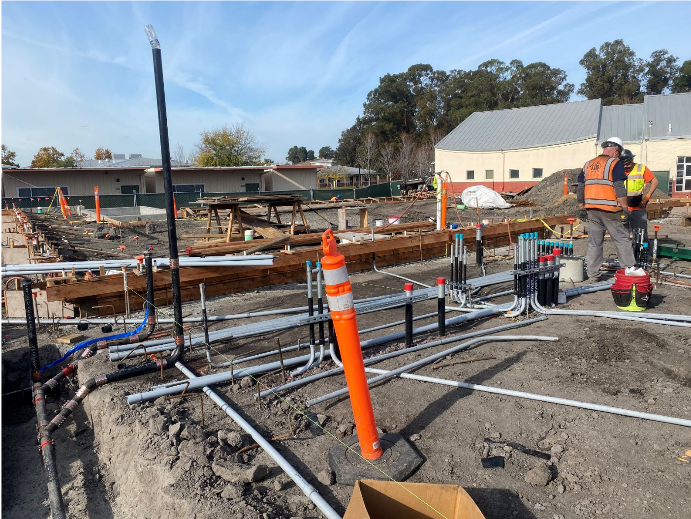
Low-voltage pathways capped into the future IDF Room
